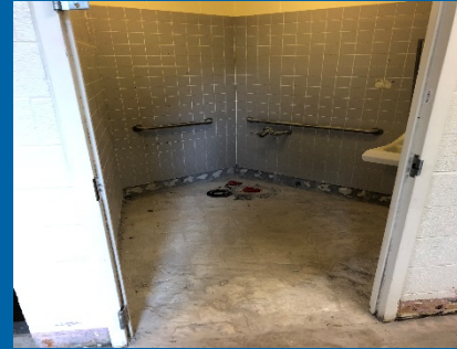
Demo of Quarry Tile Flooring and Base at Restrooms
